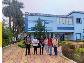
Visit to a Sewage Treatment Plant (STP) under Namami Gange Scheme, June 2022
